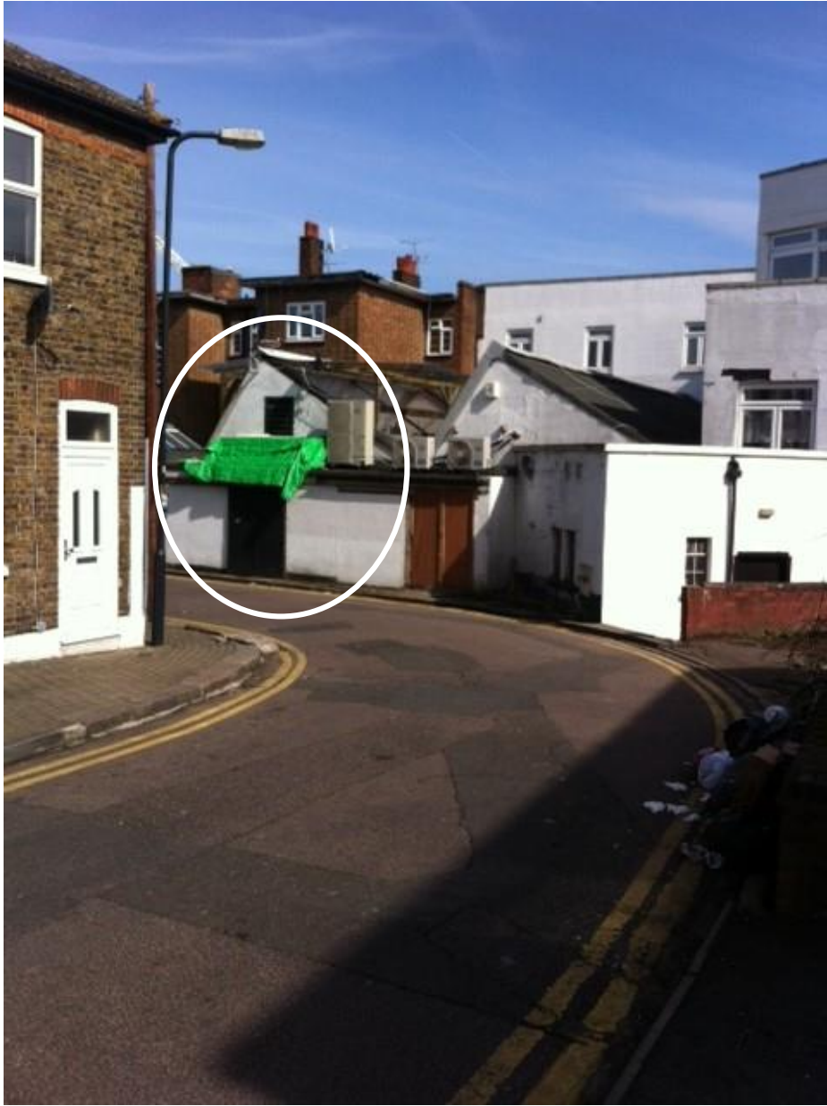
Image 1. View of rear of premises from Ecclestone Place
